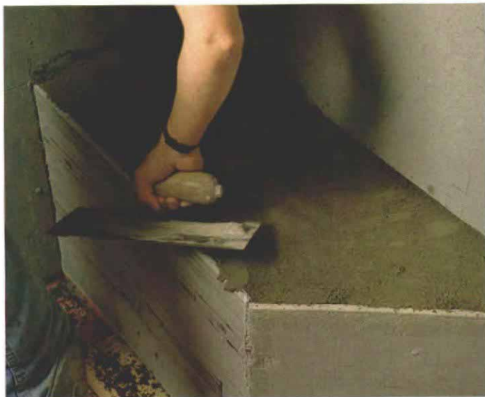
The marble for the seat goes on top of cement. The backerboard around the shower seat was left 1½ in. high, and then the resulting cavity was filled with cement, making the seat top virtually waterproof. A marble slab was used for the seat to eliminate grout joints.
