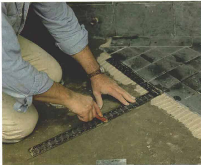
Tiling is tough on tools. A framing square is used to check the alignment of the floor tiles and to keep them running straight. But it's hard to do without plunking the tool down in fresh adhesive, which isn't great for the square.
